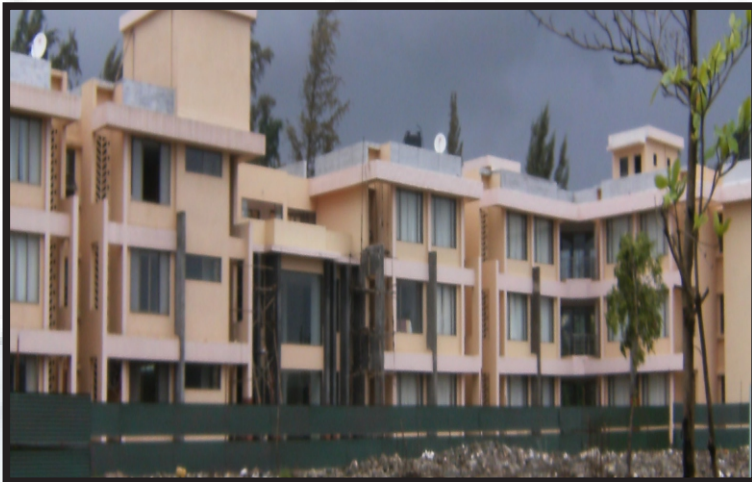
GUEST HOUSE For, DTPS - Reliance Energy
